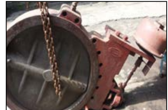
Butterfly control valve repaired and ready for use.
